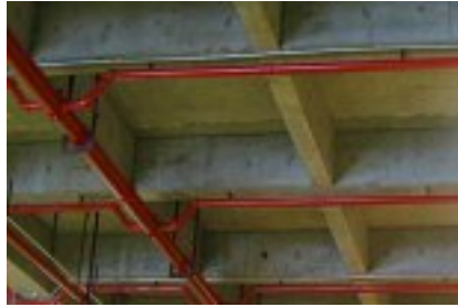
Example of an ASD pipe on the undersides of beams
