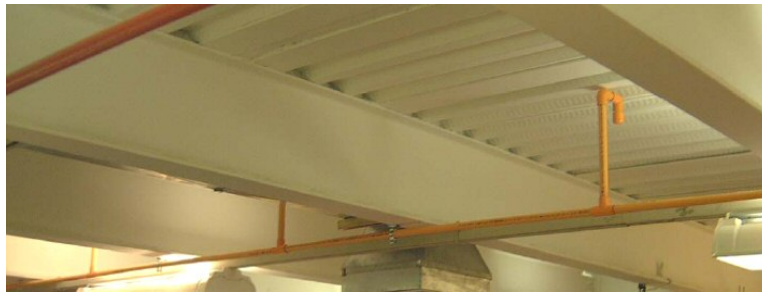
Illustration of ASD pipe sample holes extended into Inter-beam Spaces using tubes branching out from the main pipe.
