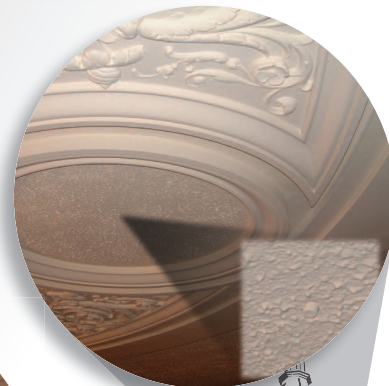
The sampling hole of the Xtralis VESDA detector can barely be seen on the ceiling of the Liberty Theatre
