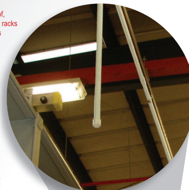
Xtralis VESDA continuously samples the air, pulling it through holes in the sampling pipes
