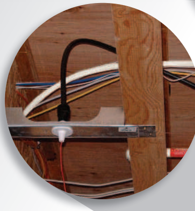
Sampling pipes can be hidden in roof spaces so that the only visible component is the tiny sampling point.
