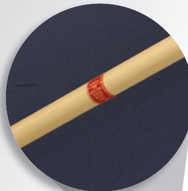
Sampling pipes installed vertically up & down walls to detect smoke stratifying below the ceiling.
